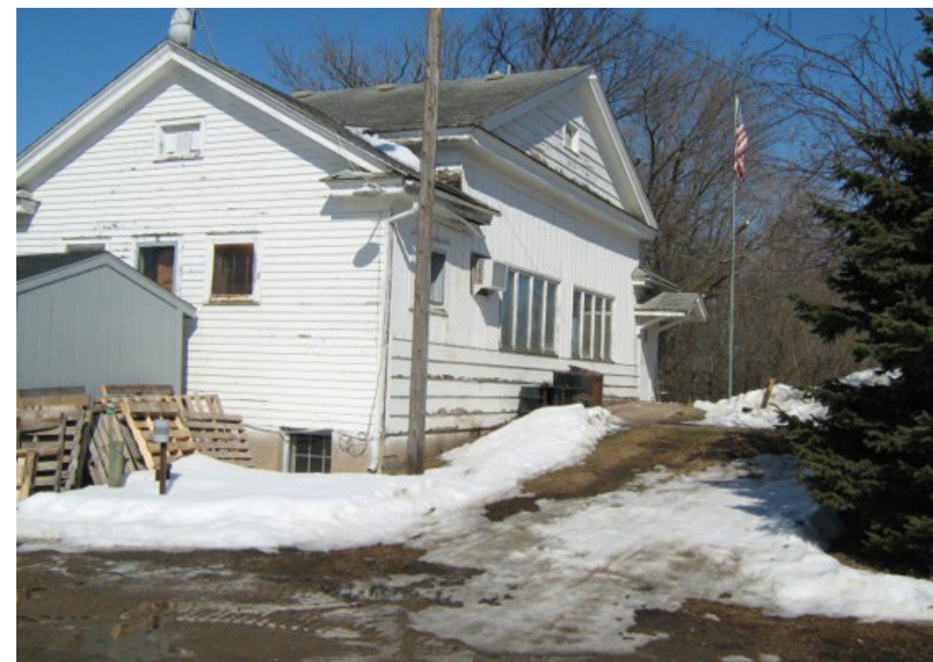
City Hall and Police Department until 1994 Continued use for Public Works until 2013
